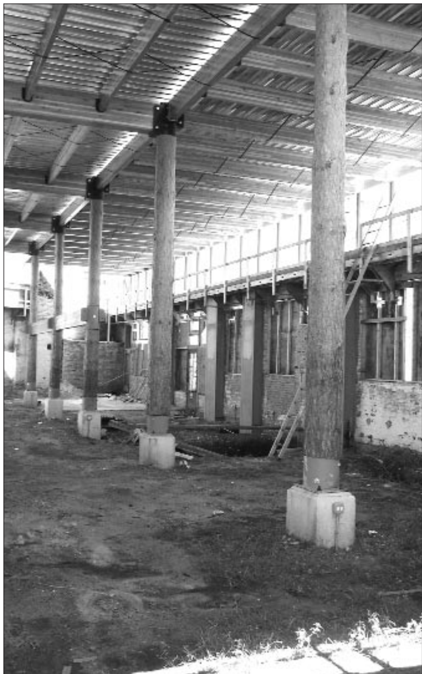
August 2004: The Experimental Station's interior under construction.
